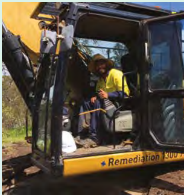
Stewart in excavator. Photo: Remondis/Kim Martin
