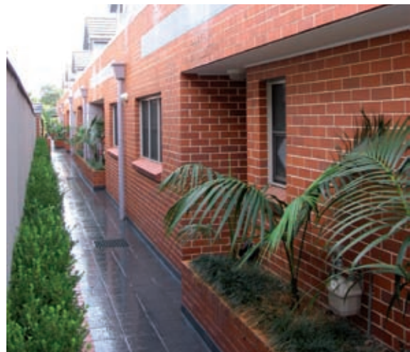
Access path for movement of bins from the storage area to and from the collection point
