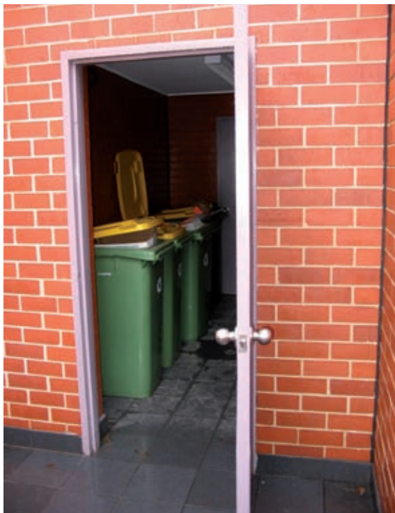
Entrance to storage area
