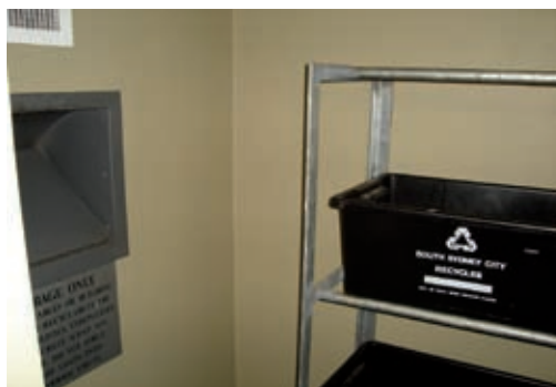
Recycling crates adjacent to garbage chute hopper
