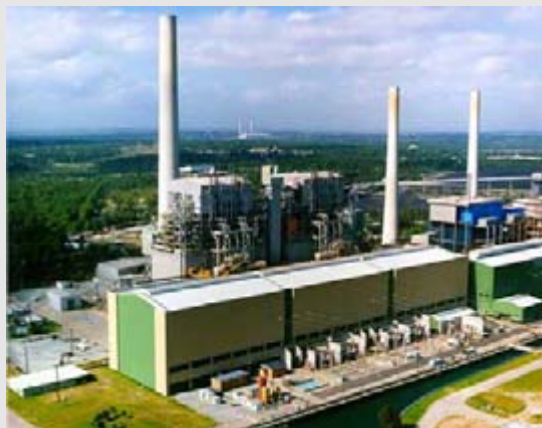
Vales Point Power Station
