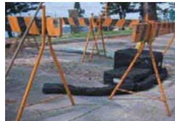
Figure 7-4 Filter bales and socks
