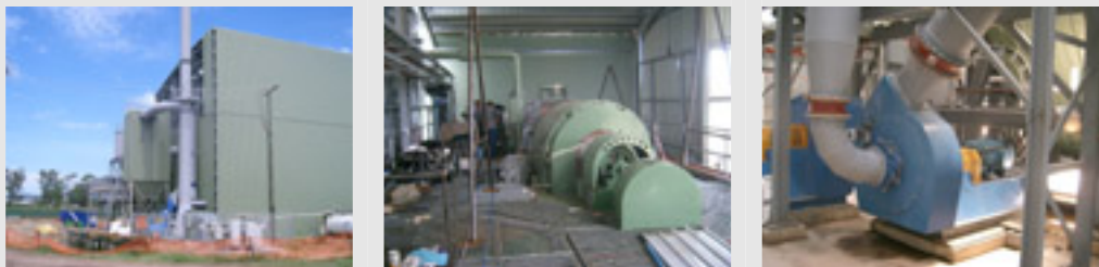
Pictures from the Staplyton Plant, Qld
