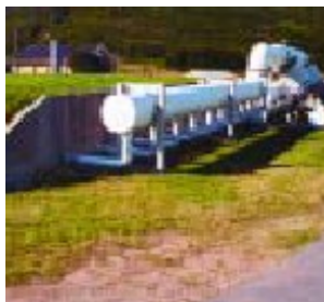
Figure 7-5 Odour biofilter at Burwood Beach Waste Water Treatment Plant
