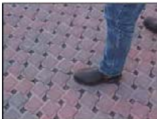
Figure 7-2 Permeable pavers, Smith St Manly
