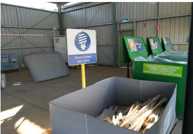
Figure 40 Sealed, well-labelled, undercover storage areas for hazardous wastes. Photo: Nicole Wilmot/EPA
