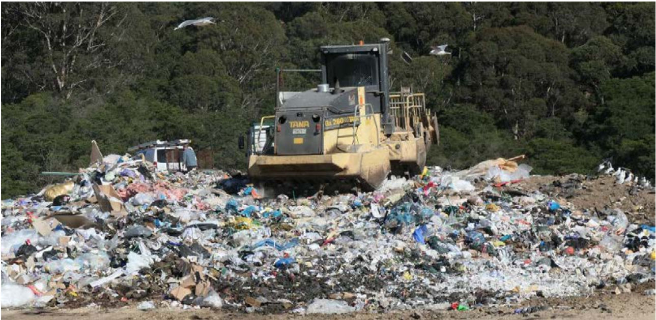
Figure 1 Waste being compacted at a landfill. Photo: Karin Schianetz/EPA
