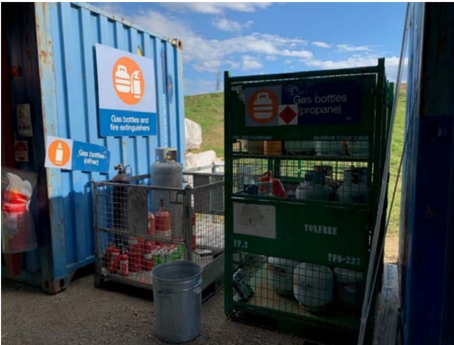
Figure 33 Safe, separate and clearly labelled storage of gas bottles. Photo: Nicole Wilmot/EPA
