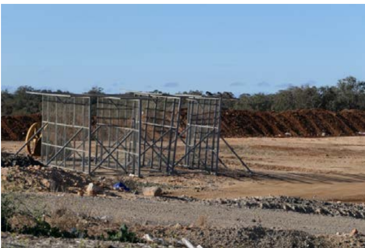
Figure 29 Additional mobile litter fencing available for use if required. Photo: Christopher Burt/EPA
