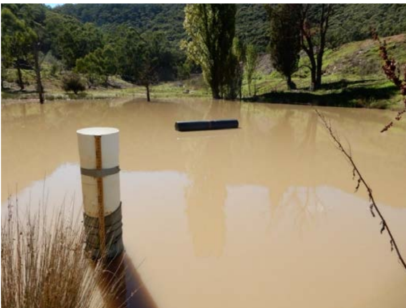
Figure 8 A sediment dam. Photo: Karin Schianetz/EPA
