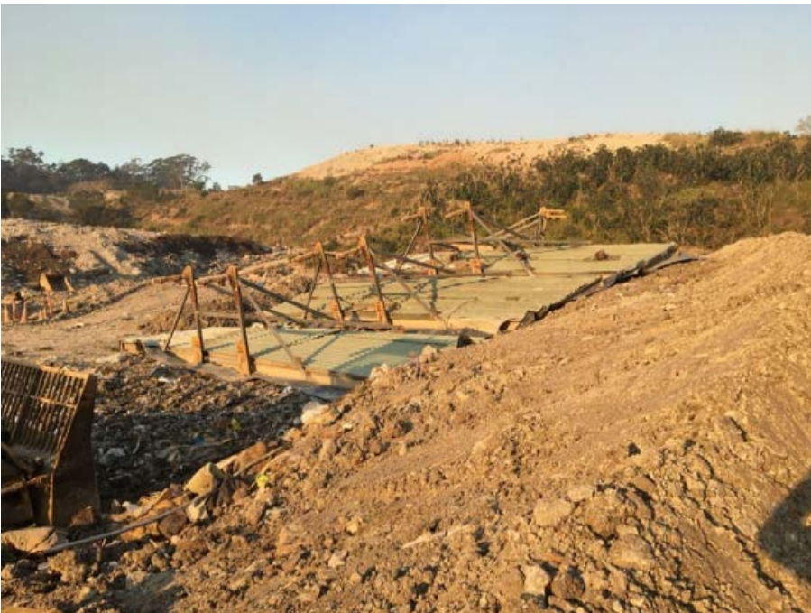
Figure 43 Proper use of landfill lids as alternative cover material. Photo: Gavin Hughes/Kempsey Shire Council
