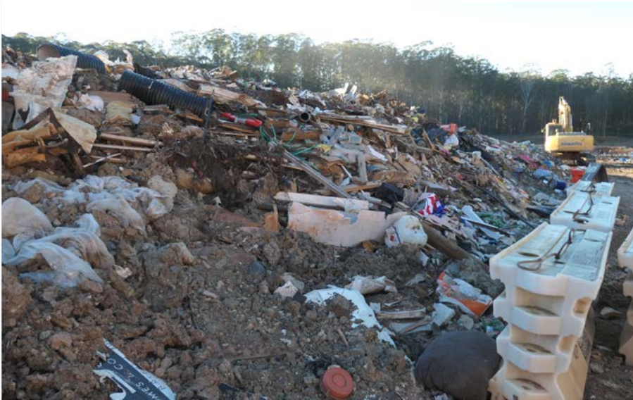
Figure 42 Large areas of waste kept uncovered. Photo: Karin Schianetz/EPA
