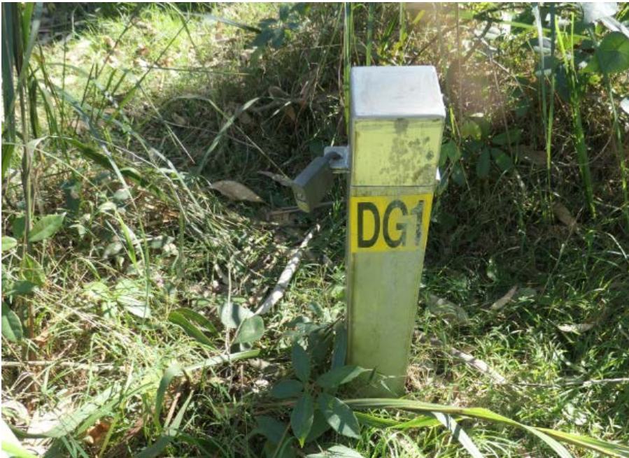
Figure 9 A groundwater monitoring bore. Photo: Karin Schianetz/EPA
