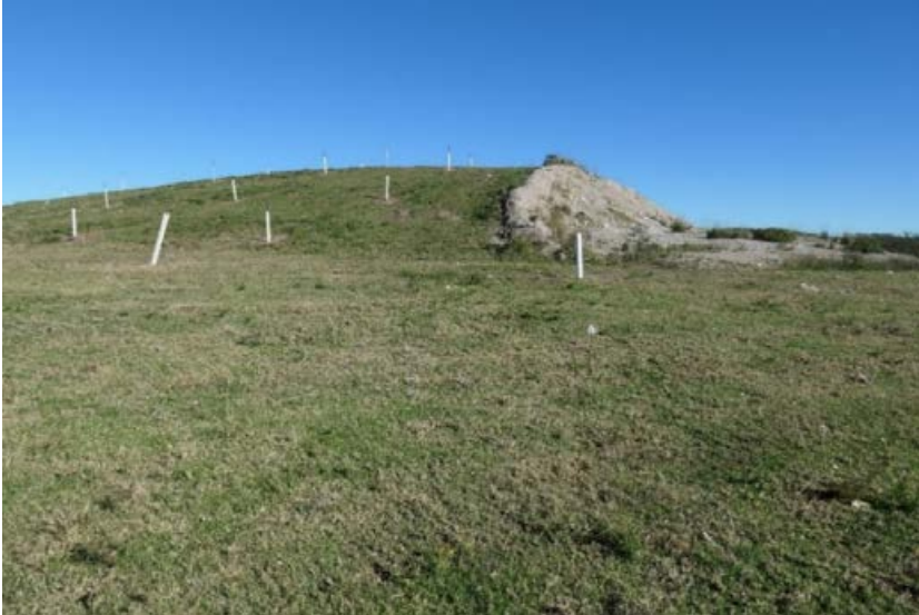
Figure 7 A capped landfill cell with irrigation. Photo: Karin Schianetz/EPA
