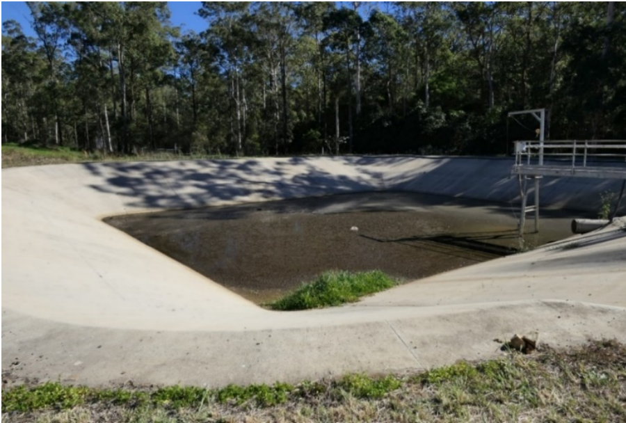
Figure 15 An emergency leachate storage basin. Photo: Lucy Silk/EPA
