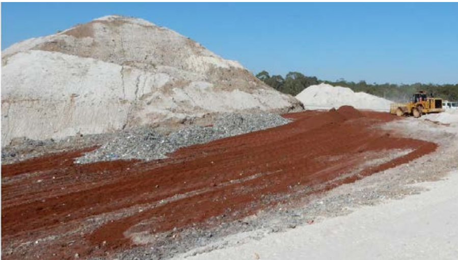
Figure 4 Covering of waste with virgin excavated natural material. Photo: Karin Schianetz/EPA
