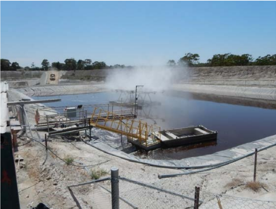
Figure 5 A leachate collection/pond with evaporator. Photo: Karin Schianetz/EPA
