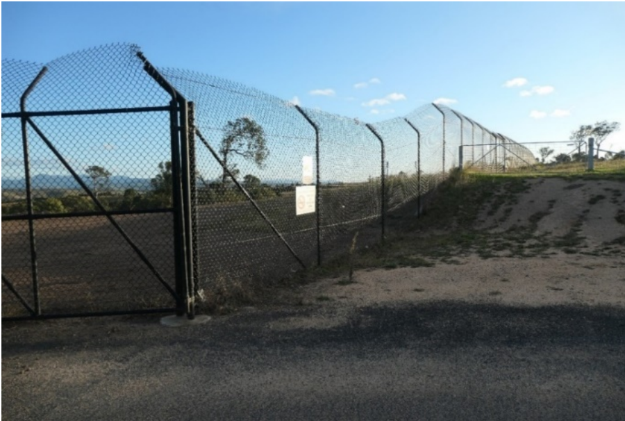
Figure 31 Stock- and wildlife-proof mesh fence around a landfill site. Photo: Karin Schianetz/EPA
