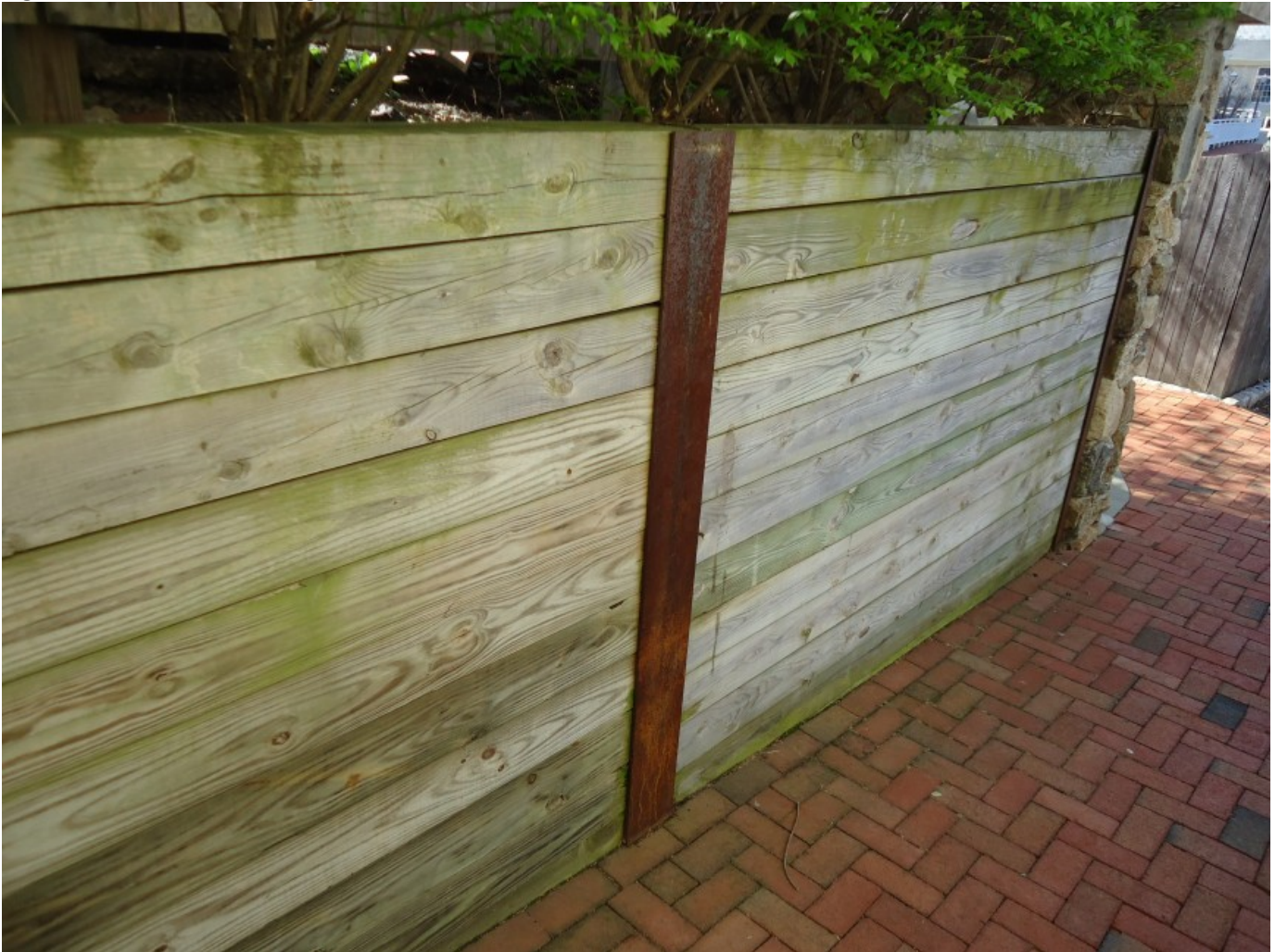
Figure 2.1. Garden retaining wall built with CCA treated timber.
