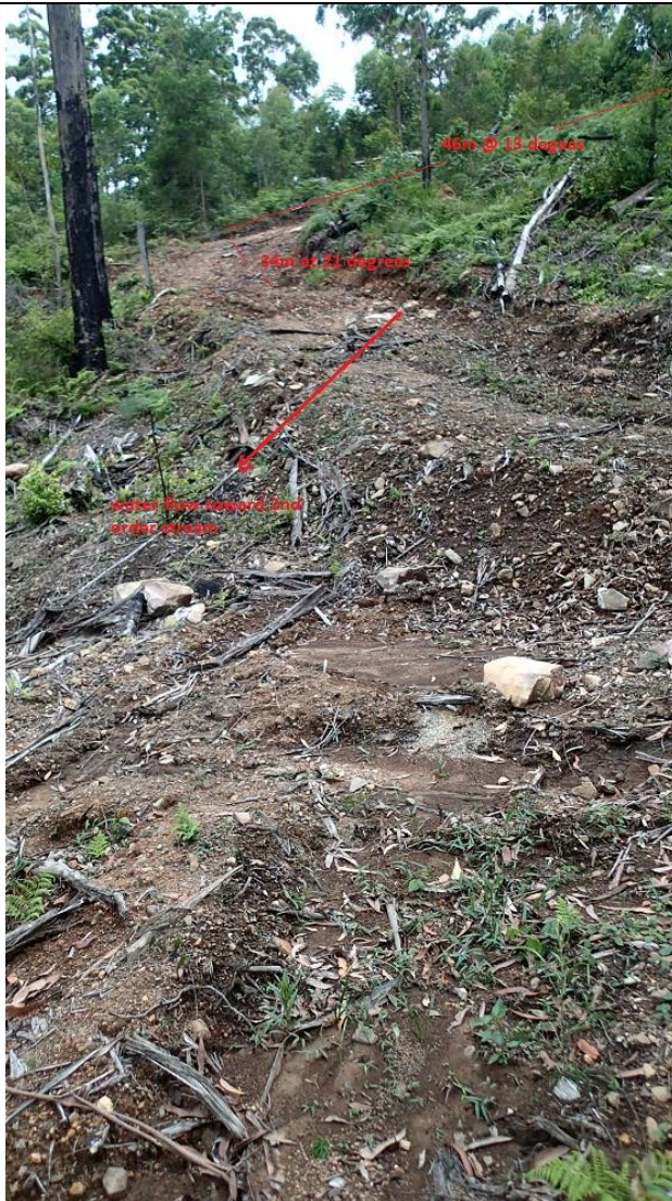
Above Snig track not properly drained (item 7)
