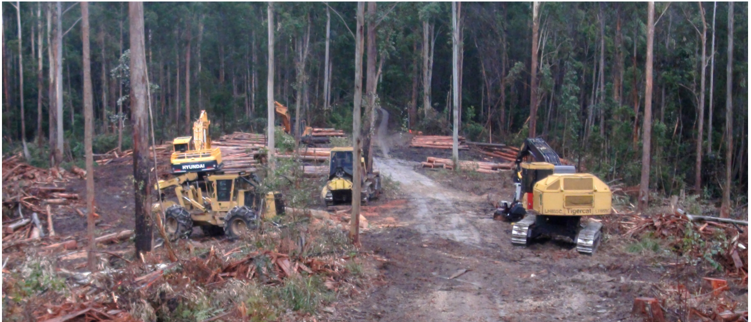
Making a start – soon all these trees will be gone
