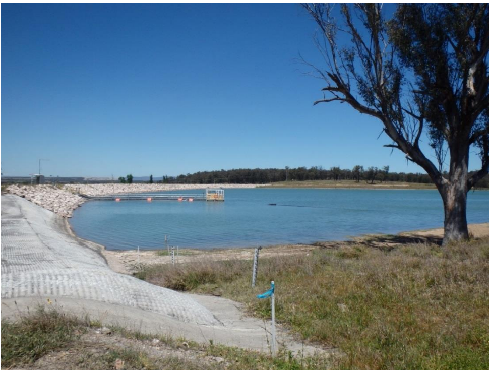
Figure 3: Wastewater holding dam for the containment of potentially saline mine water runoff (Photo: J Ehmsen/RR)
