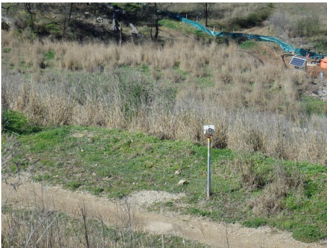
Figure 20: Example of a movement survey prism on a dam embankment (Photo: J Ehmsen/Resources Regulator)
