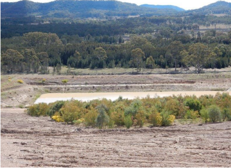
Figure 2: Sedimentation dam collecting sediment laden runoff from a partially rehabilitated area of a mine (Photo: N Wilmot/EPA)
