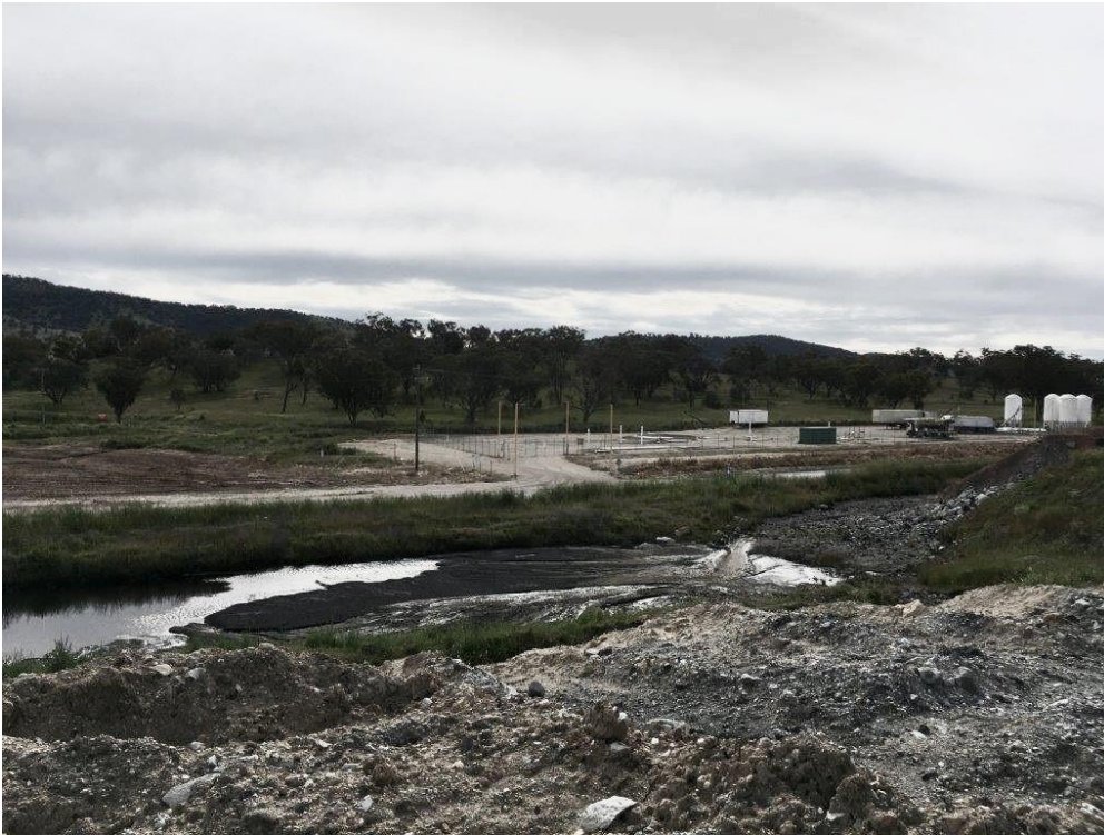
Figure 11: Sedimentation dam used to capture stormwater runoff from an area where coal stockpiles are located, resulting in coal fines and coal contact water reporting to the dam; a build-up of coal fines can be seen in the dam (Photo: E Howard/EPA)
