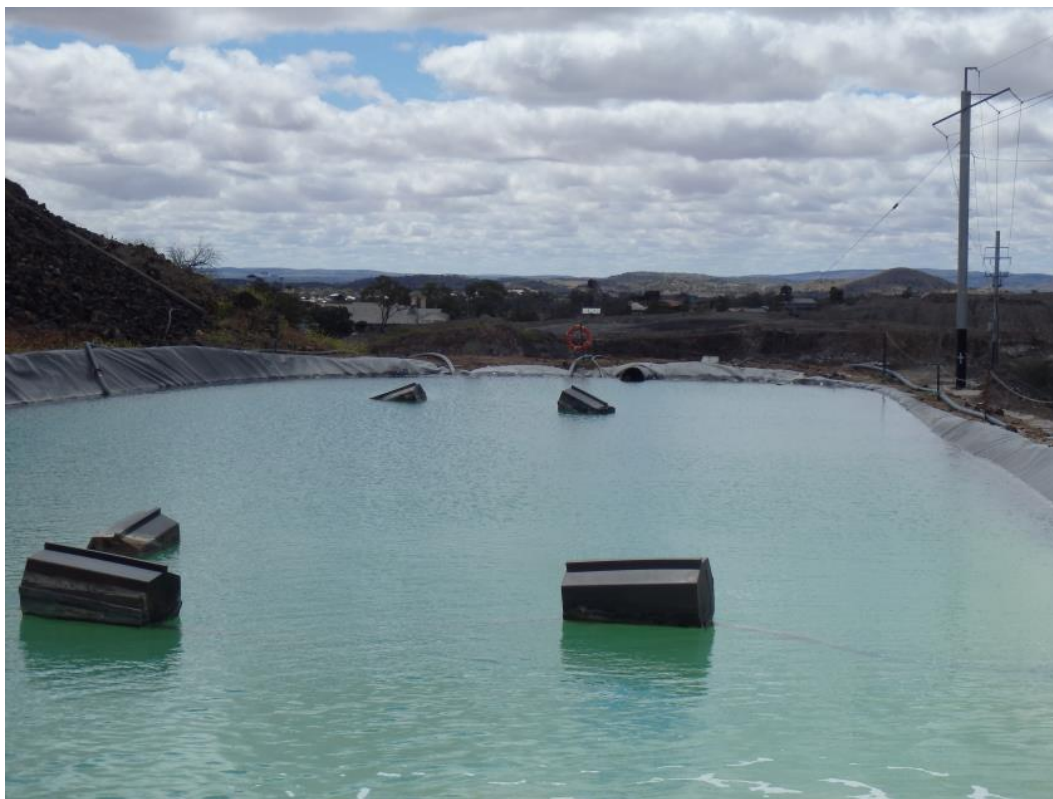
Figure 6: Inadequate dam wall construction with no operational freeboard and a noticeable low point in the dam wall (Photo: J Ehmsen/Resources Regulator)
