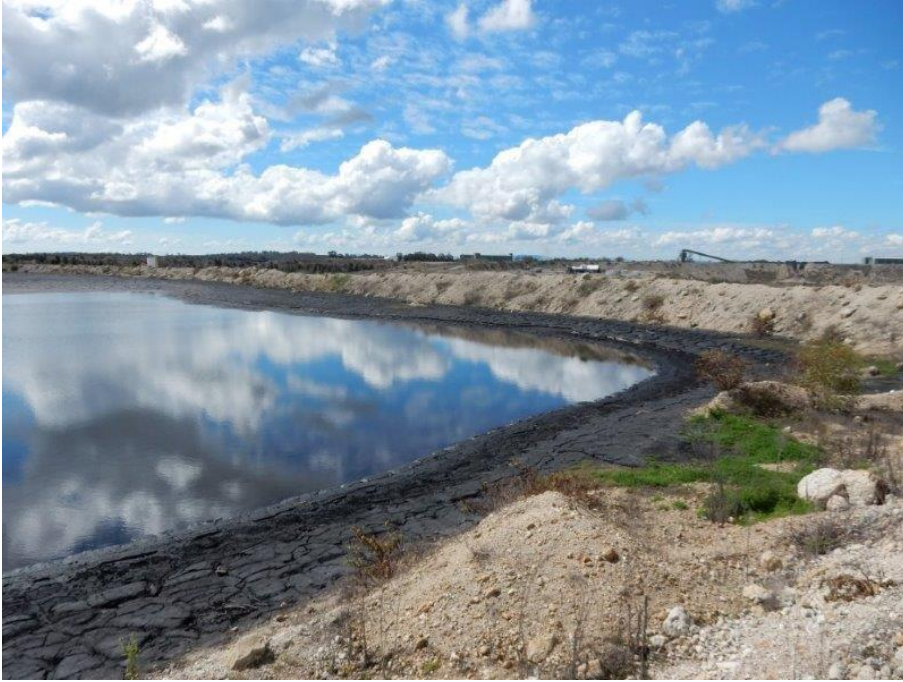
Figure 1: Storage of tailings from mining operations (Photo: N Wilmot/EPA)
