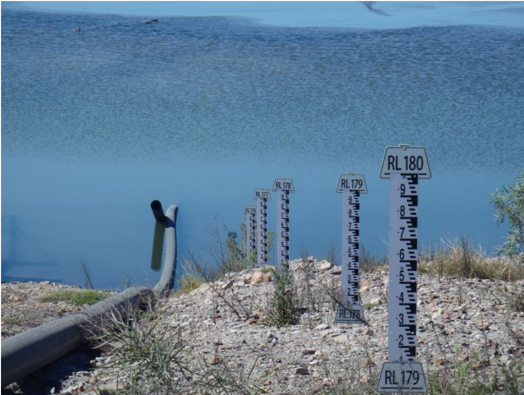
Figure 21: Example of manually read gauge marker boards in a tailings dam (Photo: J Ehmsen/Resources Regulator)
