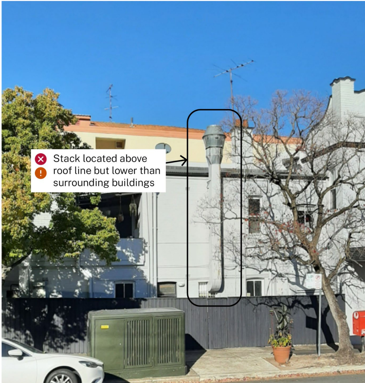
Figure 3 Stack located away from nearby buildings but below their roof levels Source: Russ Francis/Zephyr Environmental
