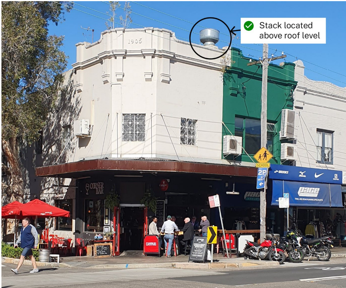
Figure 2 Well designed stack above the roof level of nearby buildings
