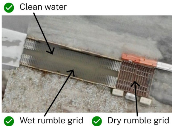
Figure 5 Effective wheel washing set-up Source: Jane Barnett/Zephyr Environmental
