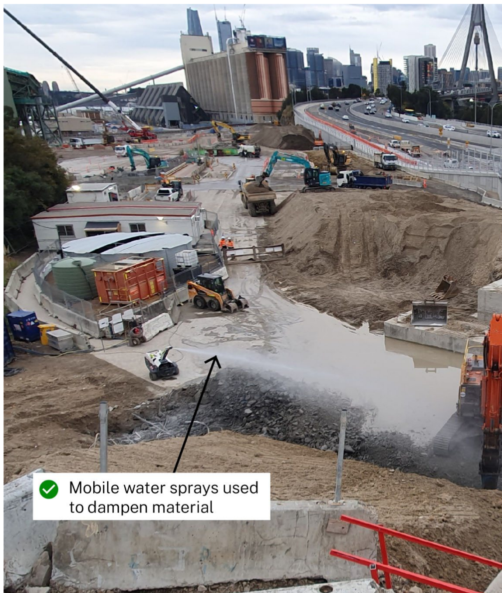
Figure 8 Mobile water spray to suppress windblown dust
