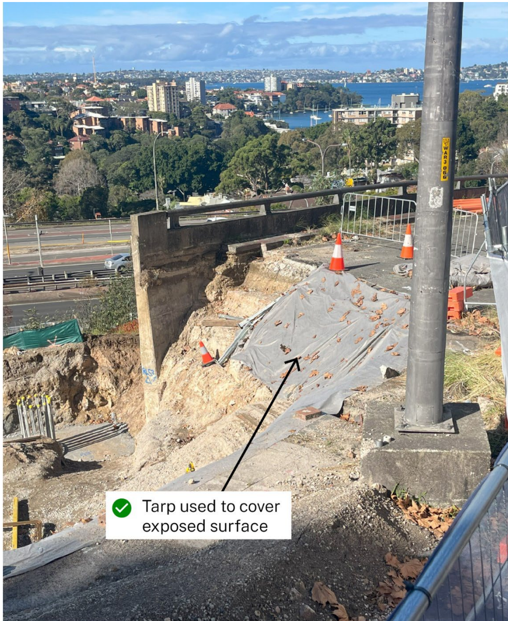
Figure 10 Tarpaulin laid over exposed surface to suppress dust
