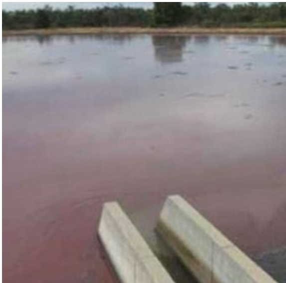
Figure 11 Well designed channel with good slope Source: APL 2015a
