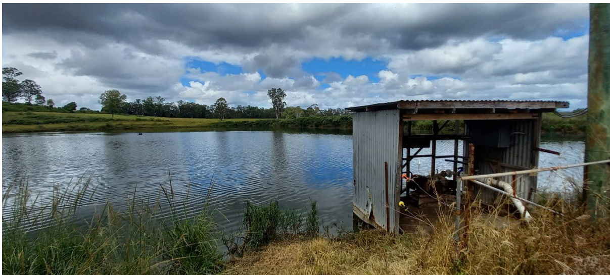
Figure 13 A well maintained effluent pond
