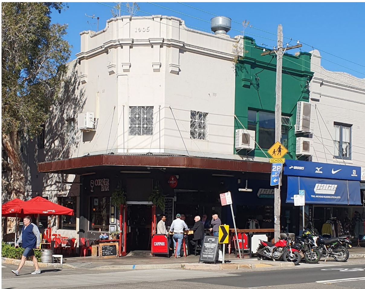
Figure 1 An appropriately designed stack may be installed for a cost comparable to an odour assessment, with a known positive outcome Source: Damon Roddis/Zephyr Environmental
