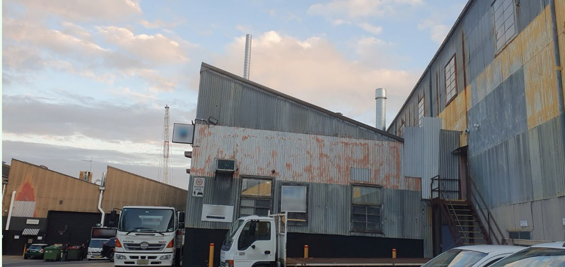
Figure 4 Craft brewery with stack showing above roofline
