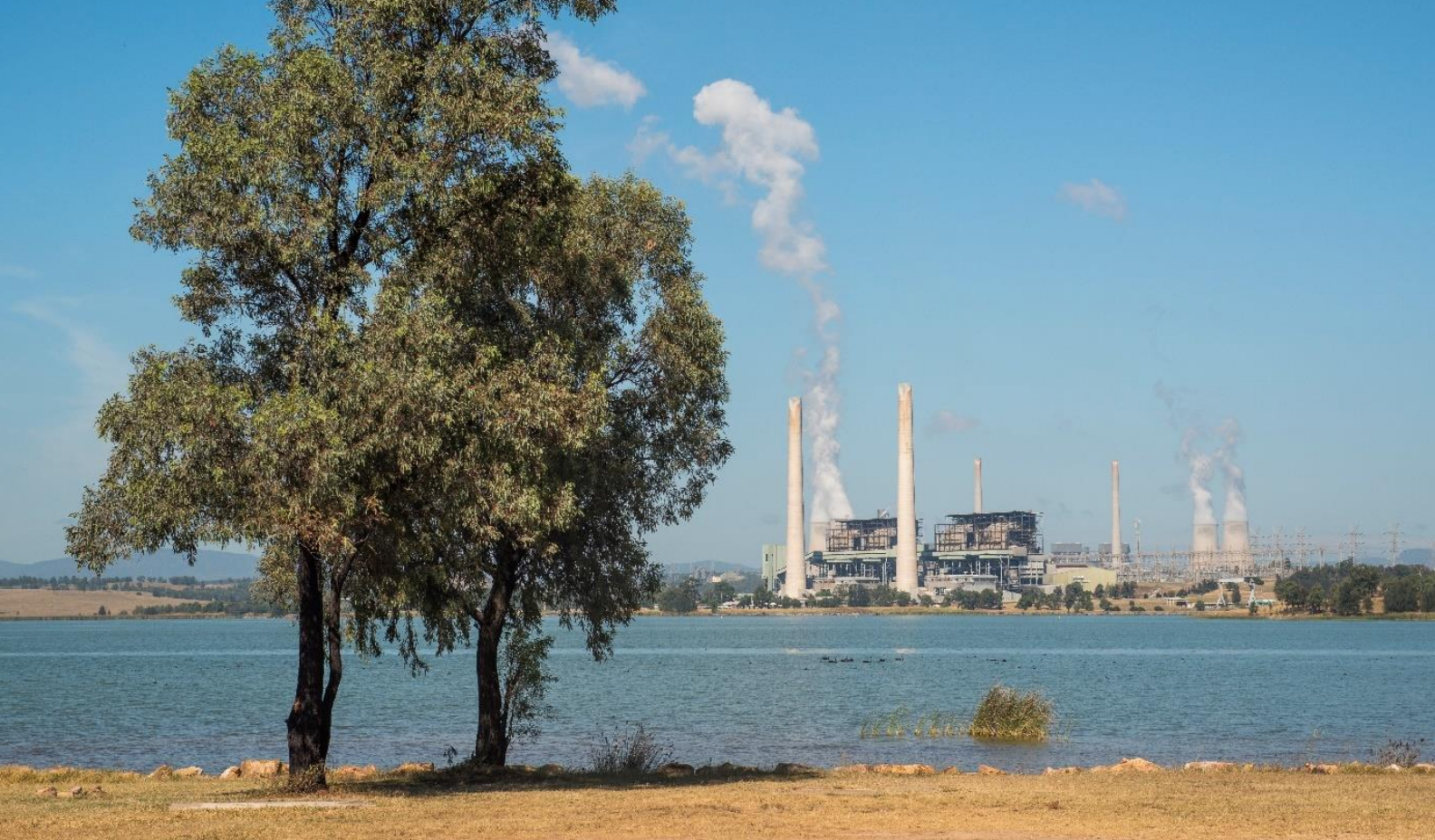
Powerplant along waterside, Muswellbrook, Wonnarua Country. Credit: John Spencer/EPA
